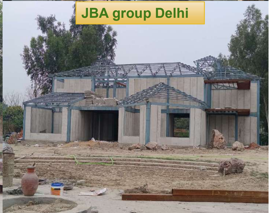
MS. structure work
